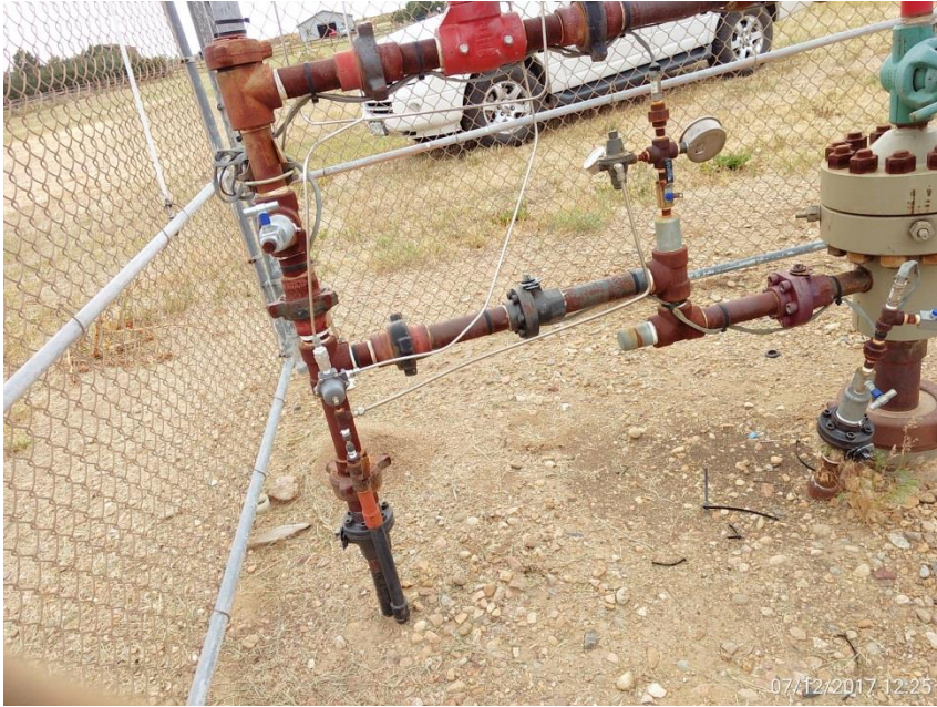
Wellhead, Note: Poly supply line point A at wellhead
