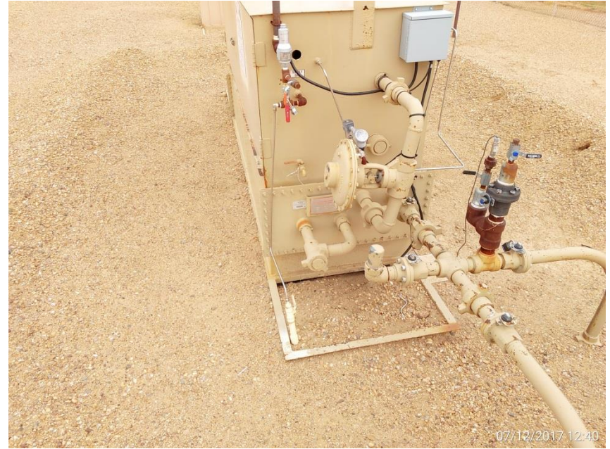
Separator, Note: Poly supply line at point B, spearator
