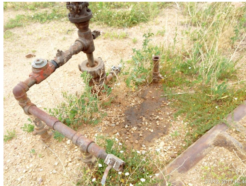
Wellhead. Corrective Action: Stained soil around wellhead
