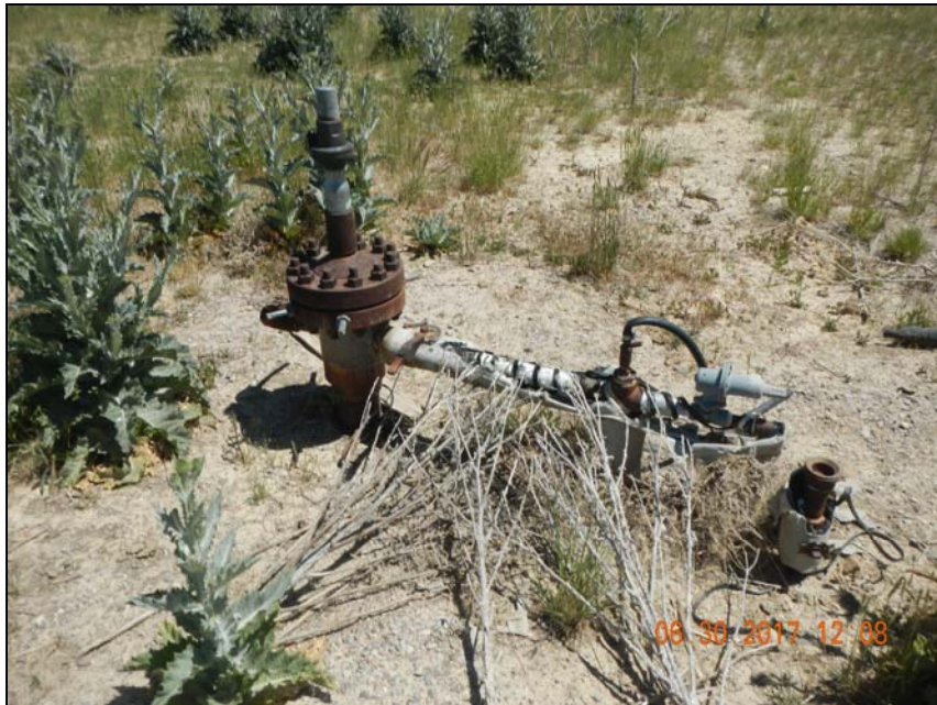
Photo 3. Risers at wellhead. Noxious weeds at wellhead. No sign at wellhead.
