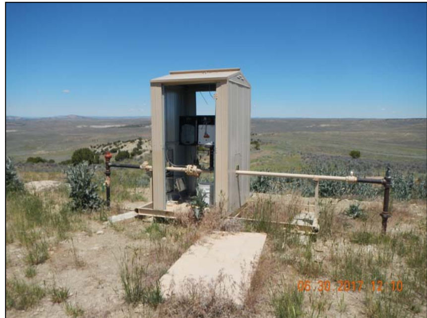
Photo 4. Meter run and risers not locked out tagged out.
