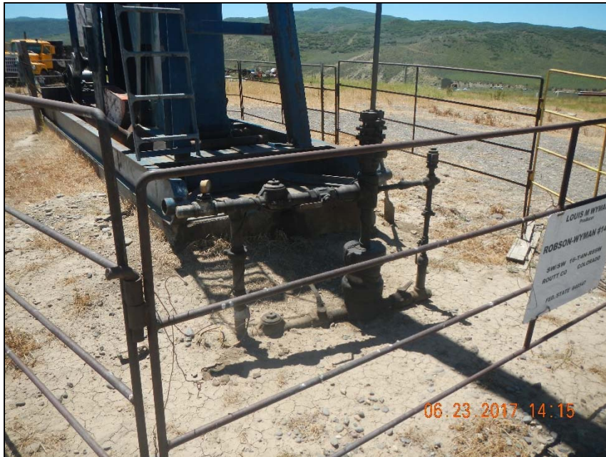
Photo 3. Risers at wellhead.
