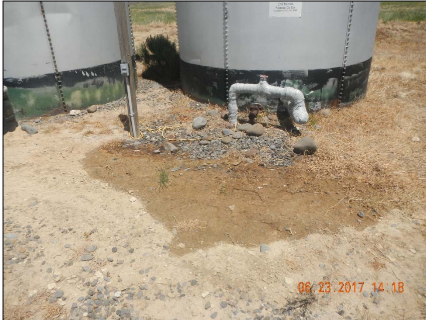
Photo 5. Stained soil in tank battery.
