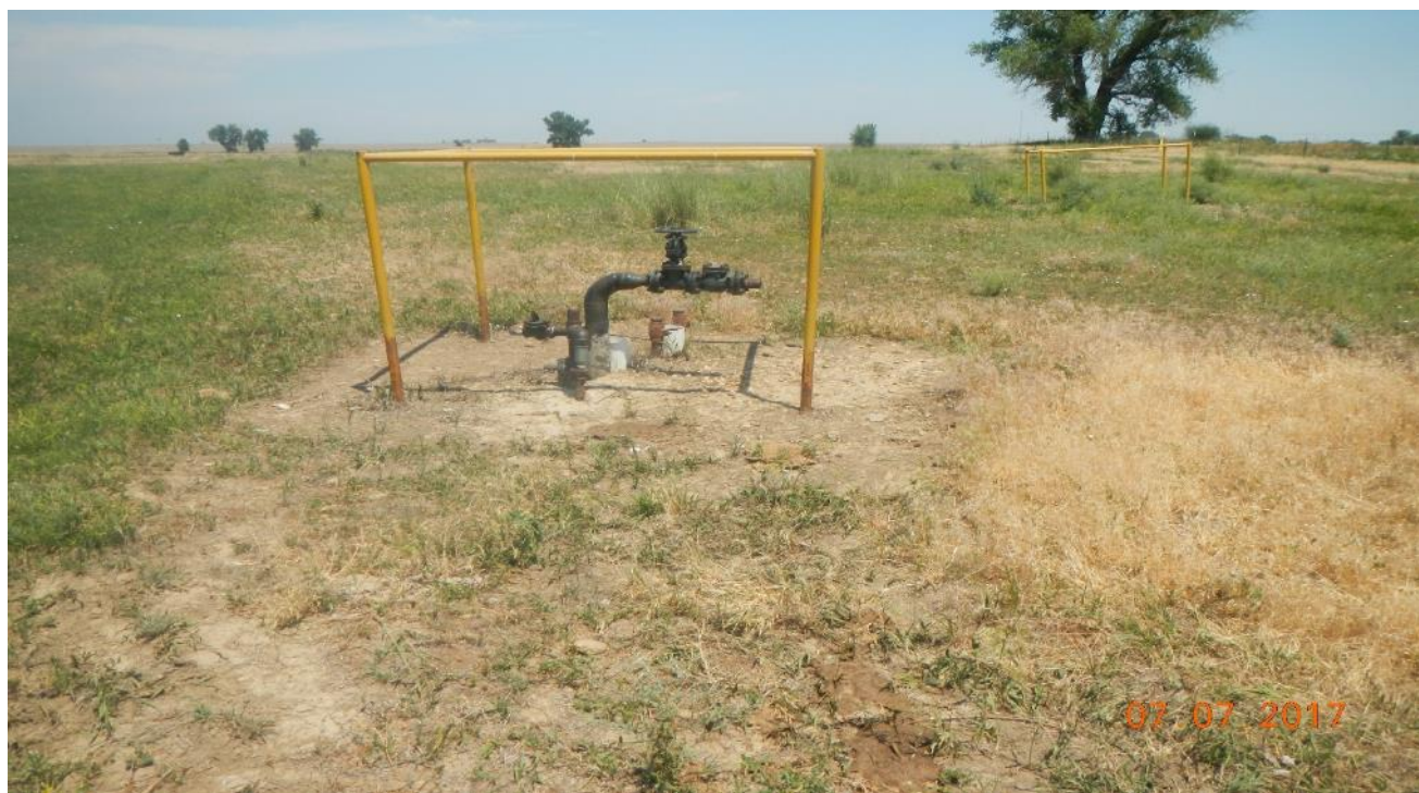
photo 2: There are pipe risers that remain at the tank battery site. Lat/Long:40.03149,-104.91935
