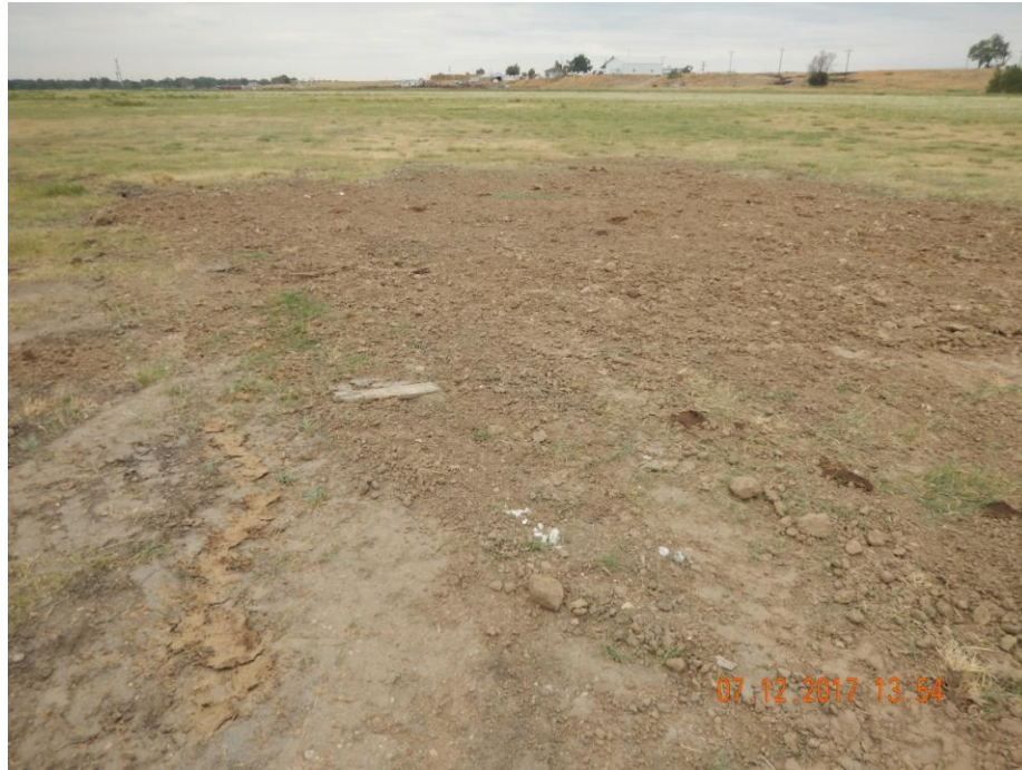
Photo 1: Photo taken from the well location, facing east. Photo shows well has been plugged and removed. If compaction alleviation has not yet been performed, well will require cross ripping as well as revegetating to reflect the adjacent reference area.
