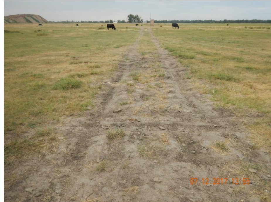
Photo 2: Photo taken from the well location, facing north. Photo shows access road has yet to be reclaimed. Access road appears to require compaction alleviation, re-contouring, re-grading and re-vegetation. Reclamation rule 1004.a requires all such reclamation work be completed within twelve (12) months on non-crop land after plugging a well.
