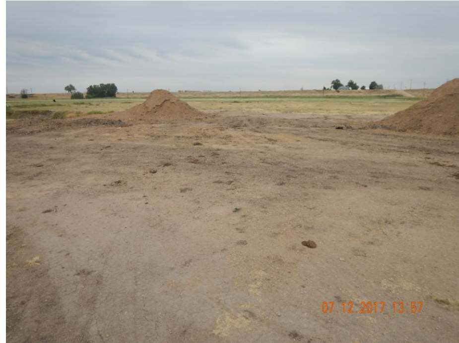
Photo 5: Photo taken from the north end of the battery location, facing south west. Photo shows equipment at the battery facility have been removed. Battery location waiting additional reclamation activities; location appears to still require road base removal, compactions alleviation, re-contouring, re-grading and re-vegetation. Reclamation rule 1004.a requires all such reclamation work be completed within twelve (12) months on non-crop land after plugging a well.
