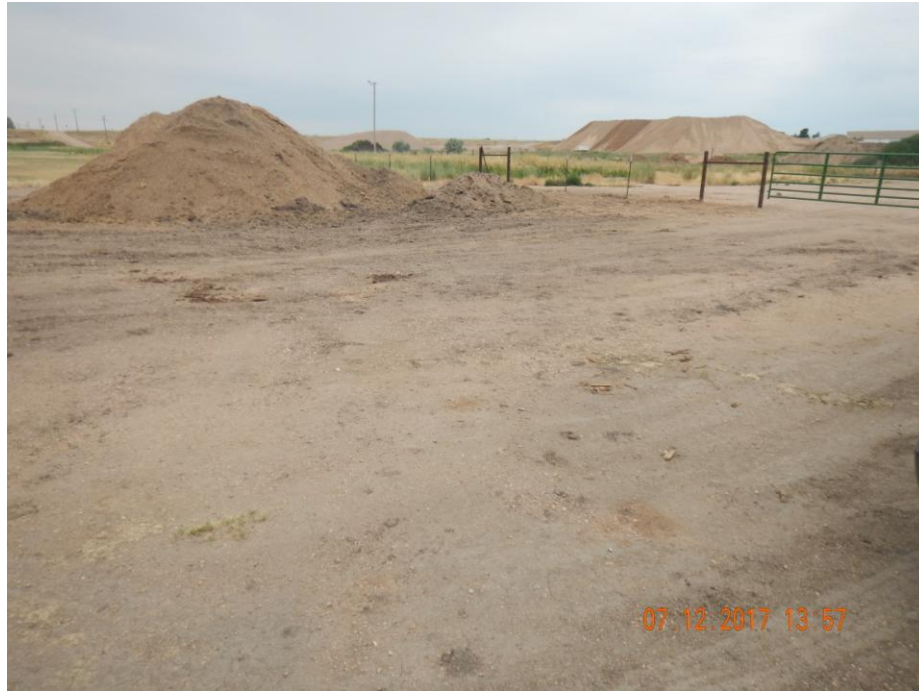
Photo 4: Photo taken from the north end of the battery location, facing south west. Photo shows equipment at the battery facility have been removed. Battery location waiting additional reclamation activities; location appears to still require road base removal, compactions alleviation, re-contouring, re-grading and re-vegetation. Reclamation rule 1004.a requires all such reclamation work be completed within twelve (12) months on non-crop land after plugging a well.
