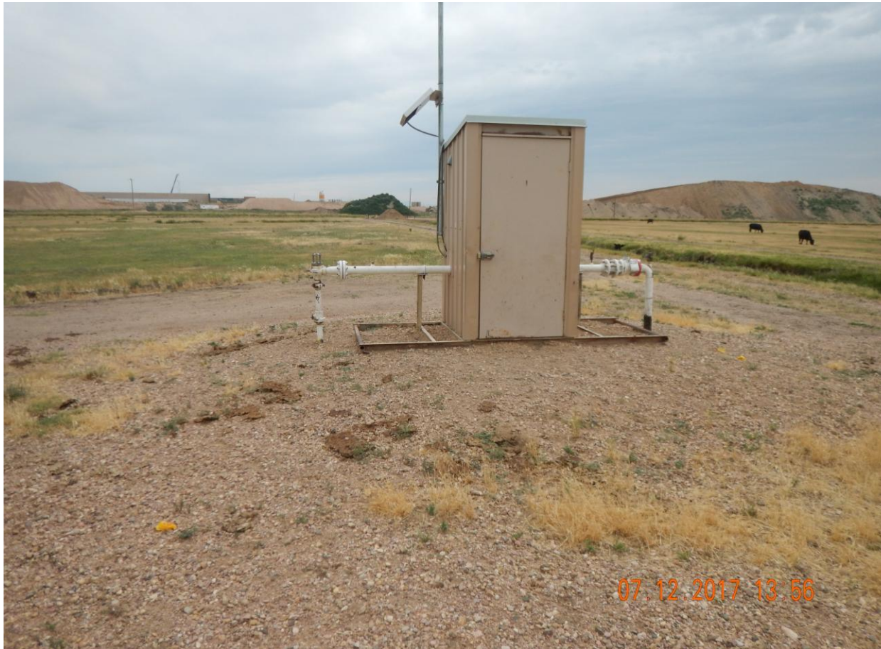
Photo 3: Photo taken from the north of the well location, facing west. Photo shows meter shed that has not been removed. Reclamation rule 1004.a requires that all equipment be removed within three months of plugging the associated facility.
