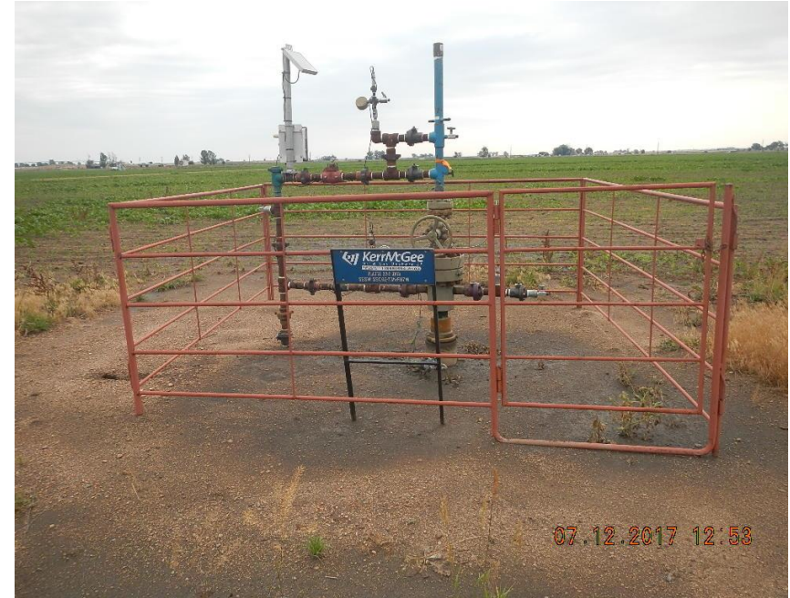
Photo 2 Wellhead from west
