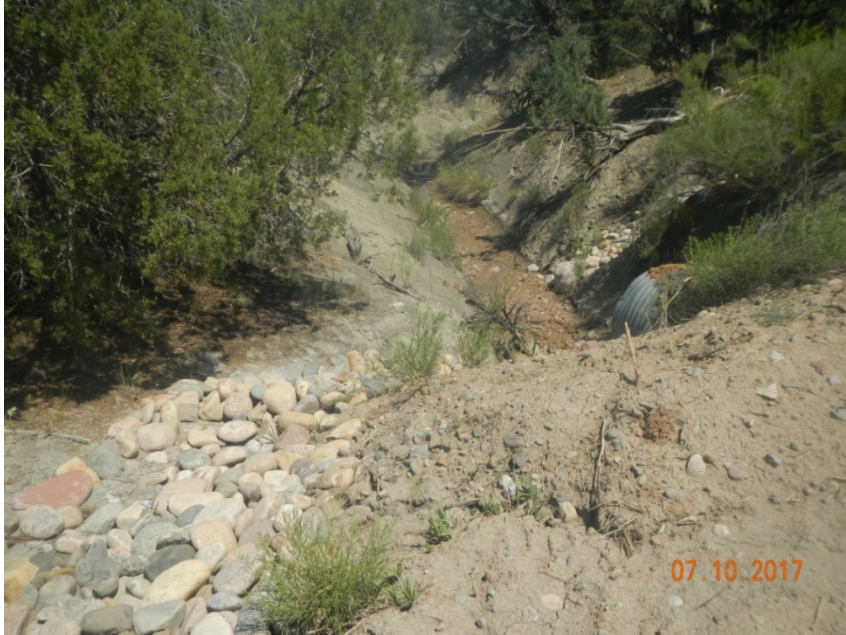
Photo 1: View of cobble run-down installed along the southern edge of culvert along access.
