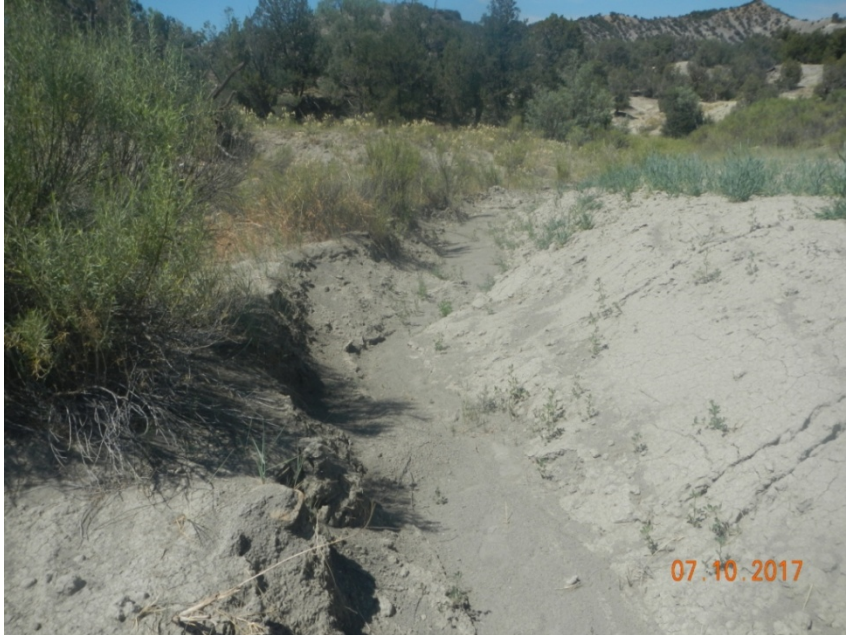
Photo 5: View of sediment filled diversion along the southeastern edge of the project area facing downstream (southwestward). Stormwater controls are needed to stabilize sediment transport in this area.
