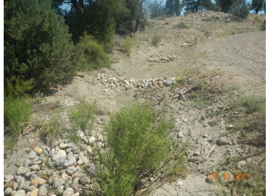
Photo 2: View of cobble run-down and check dams along roadside drainage north of culvert shown in Photo 1.
