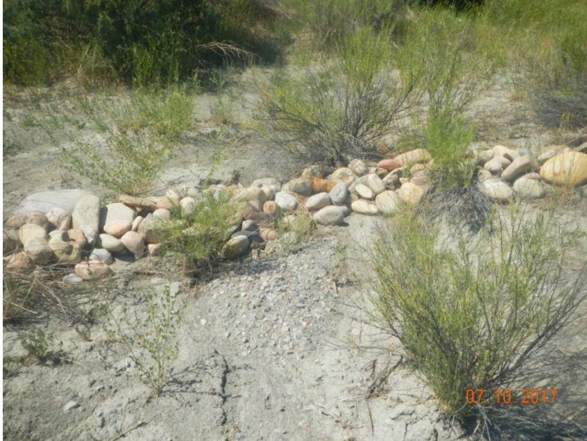
Photo 3: View cobble check dam in the southeastern portion of the project area. Appears to be installed to filter flows off of the southern portion of the well pad.
