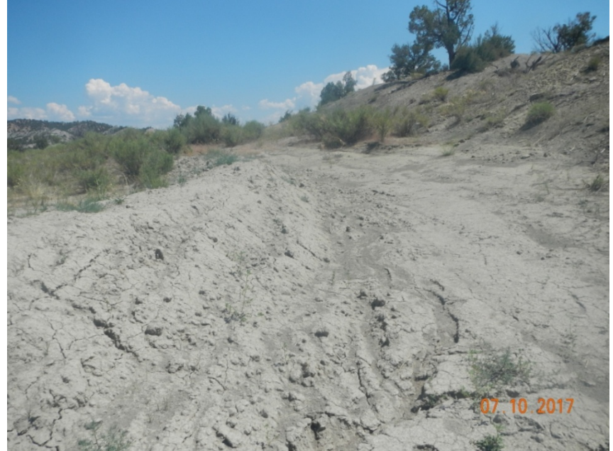
Photo 6: View of sediment filled diversion with exposed soils and no stormwater controls, facing upstream (northward). Stormwater controls are needed to stabilize sediment transport in this area.
