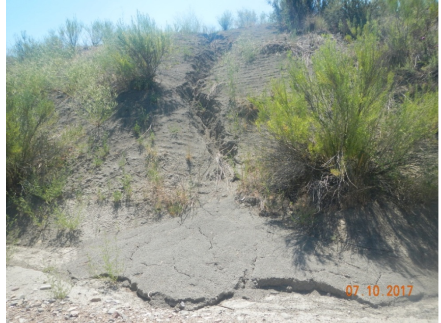
Photo 8: View of erosion in the northwestern fill slope, depositing sediment onto the access road and into the flow pattern of roadside drainage.
