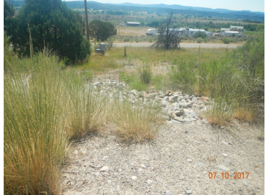
Photo 2: View of cobble run-down installed since the December 2016 reclamation inspection. Appears to be functioning.
