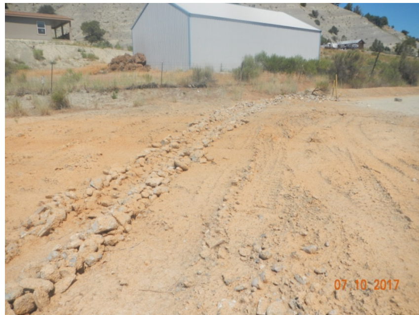
Photo 4: View of newly installed cobble-lined diversion in the southwestern portion of the project area. Appears to be functioning.
