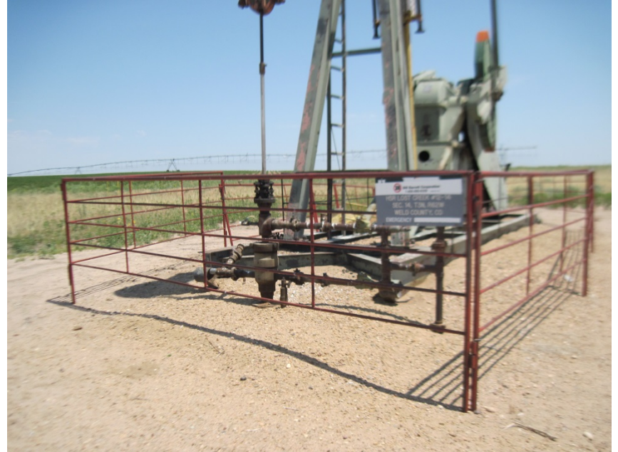
PUMP JACK AND WELLHEAD
