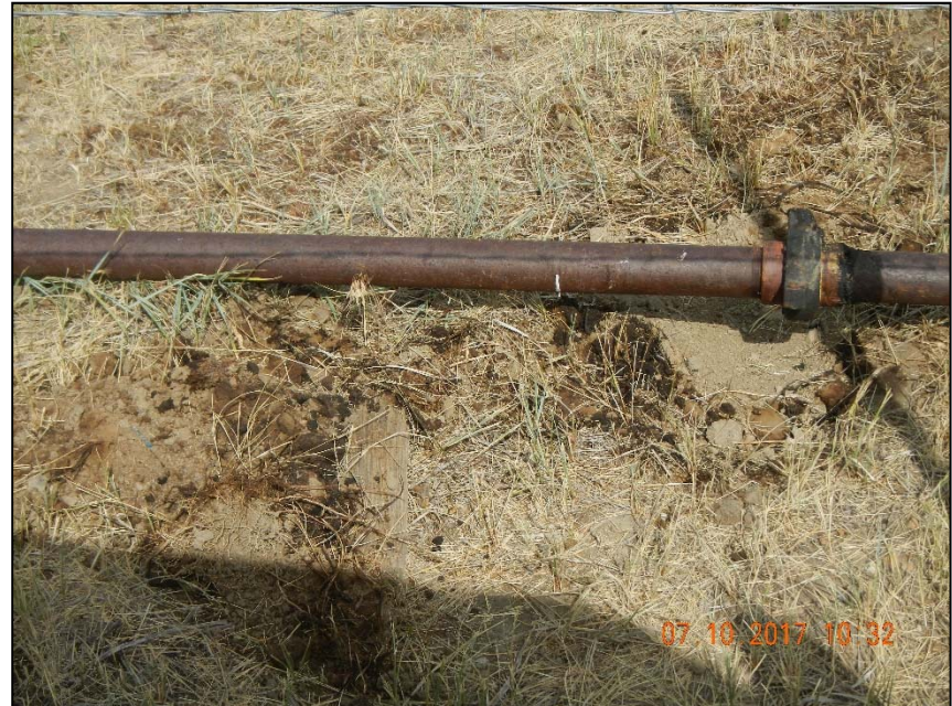
Photo 4. Close-up of leak and clean-up efforts at threads.
