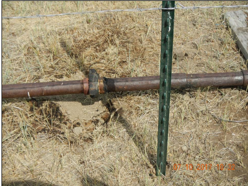
Photo 5. Close-up of leak and clean-up efforts at threads.
