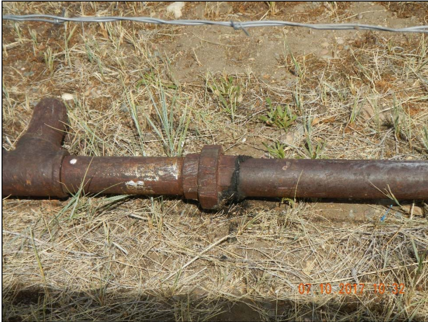
Photo 3. Close-up of leak remaining at threads.
