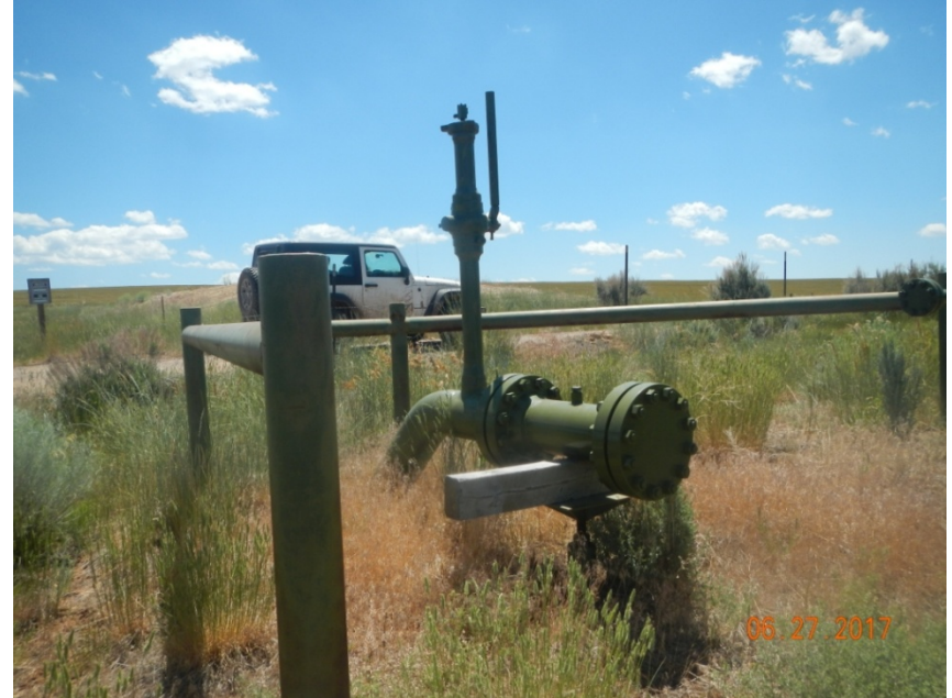
Photo 2: View of riser at 37.53328, -108.62963, across county road entrance to project area. Lockout/tagout not observed.
