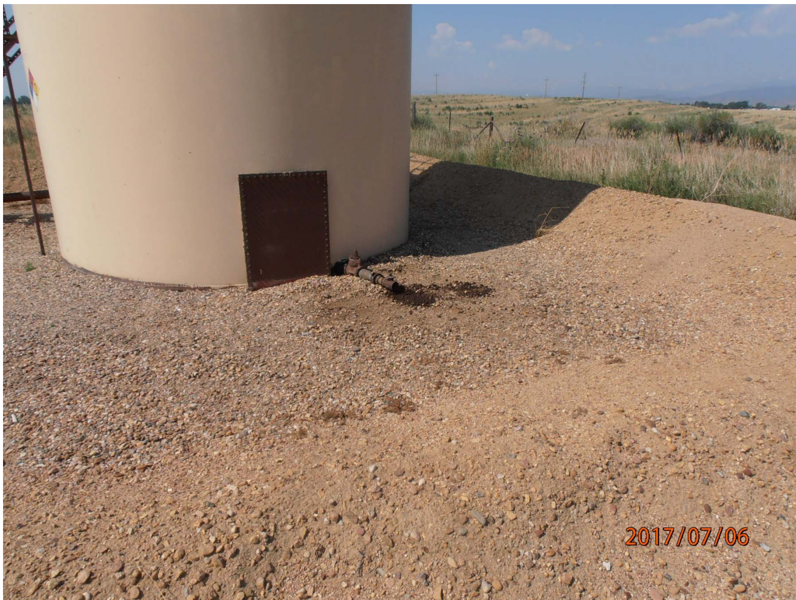
Leaking crude oil AST valve north side of tank.
