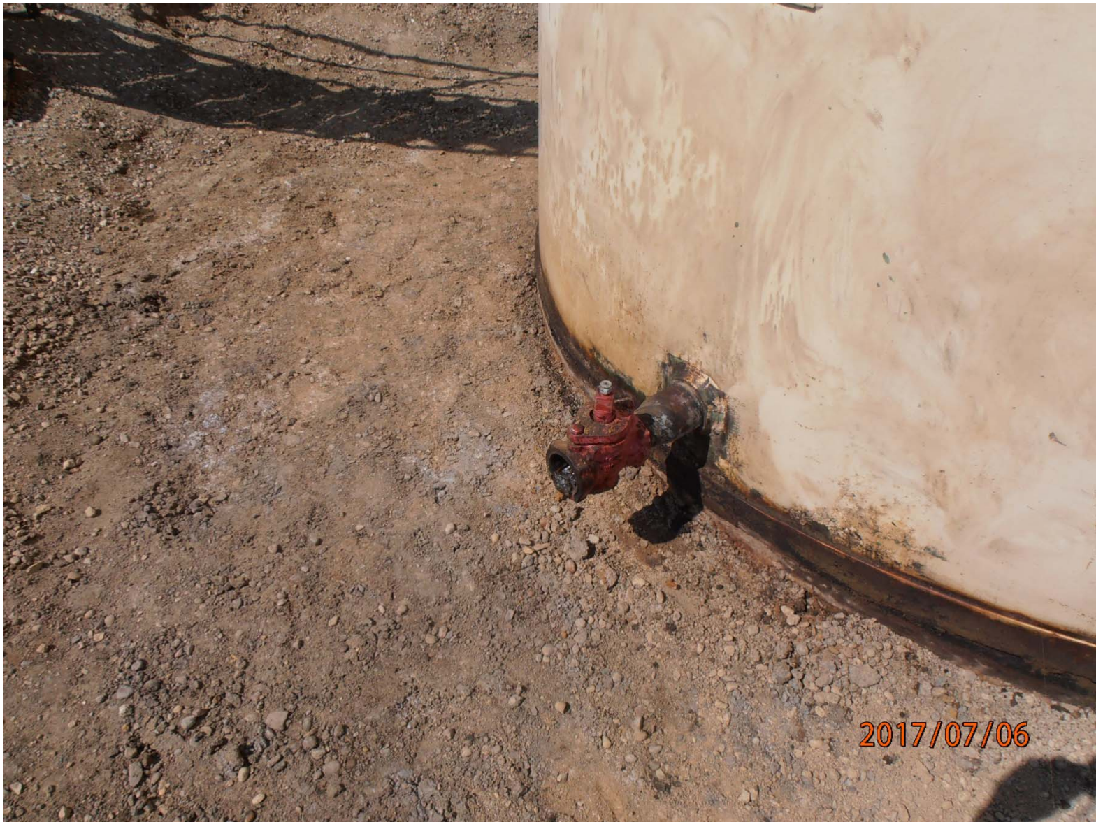
Valve on produced water AST.
