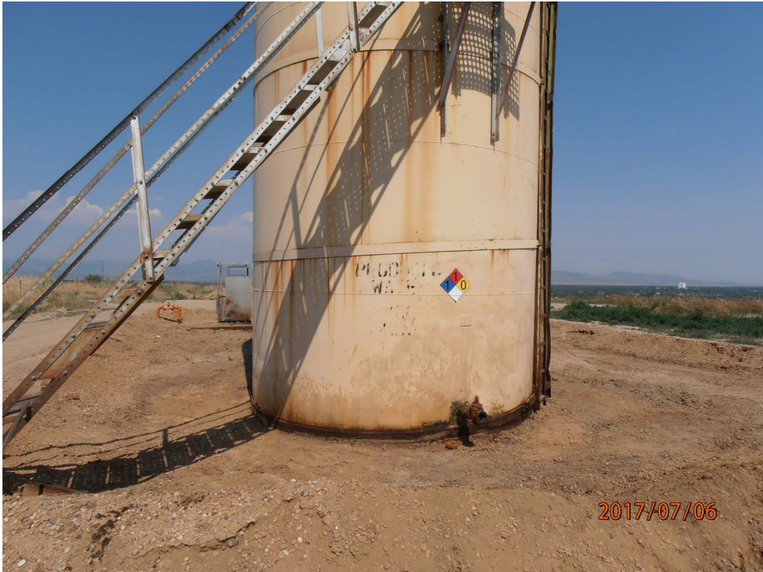
Produced water AST lacks contents, capacity and operator information.
