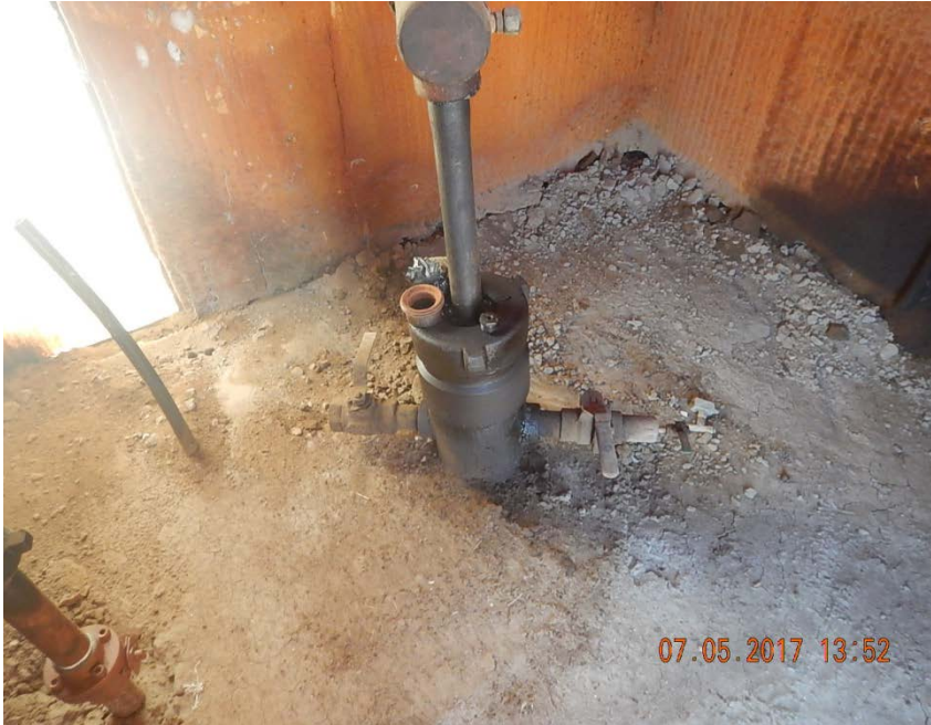
Photo 1: No bradenhead at surface
