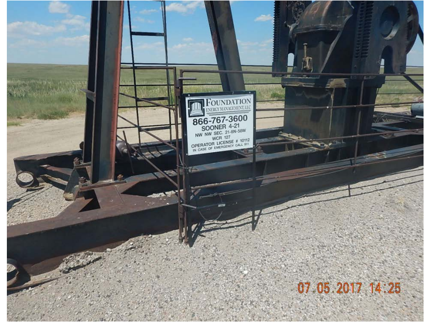
Photo 1: Wellhead sign at well
