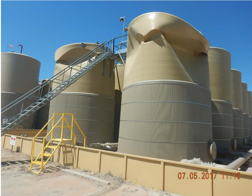
Photo 2: Damaged tanks at battery.
