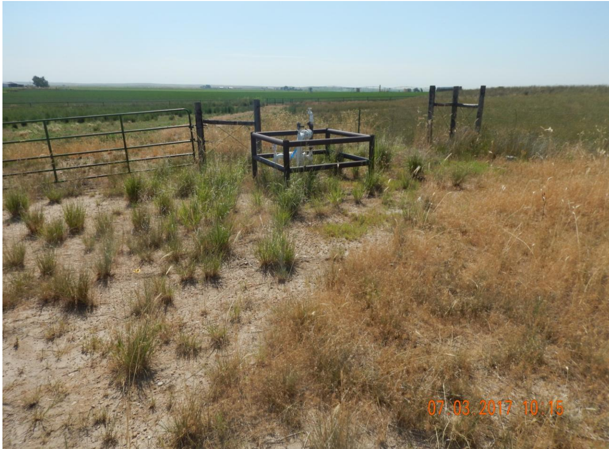
Photo 1: Photo taken from the southeast corner of the battery location, facing southeast. Inspection doc. # 682401398 required operator to remove risers from battery location. Photo shows risers have not been removed.
