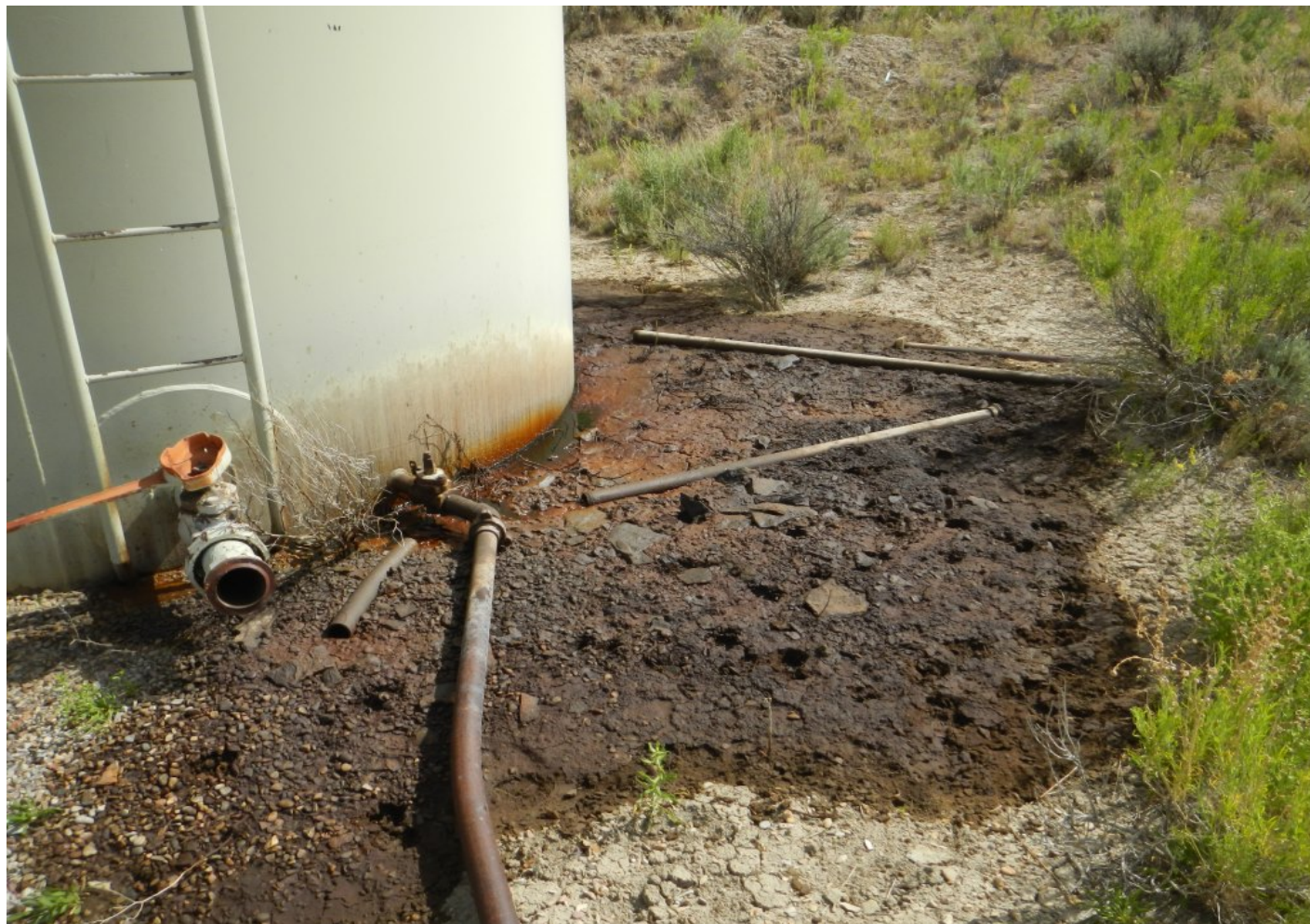
Photo#2: Tank #1, rusted at base & leaking.
