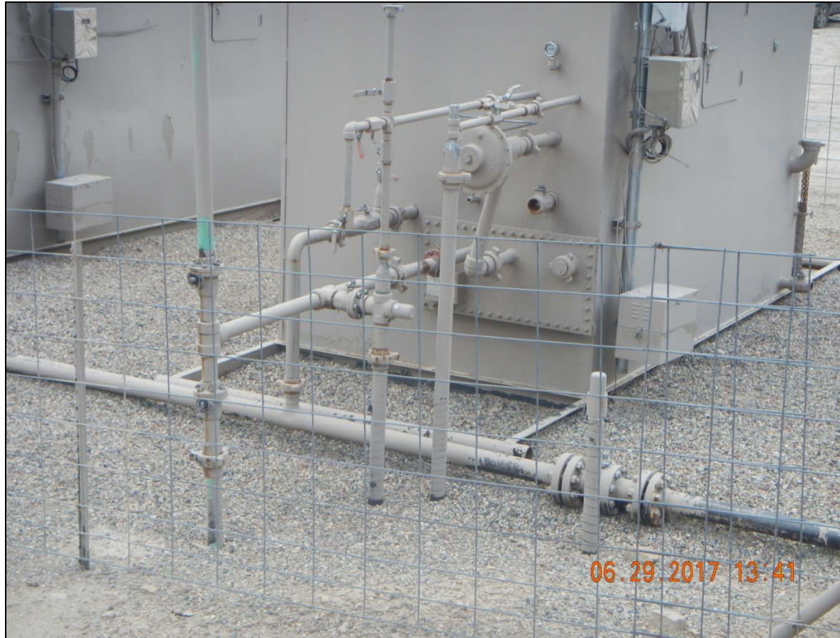
Unused riser at separators.
