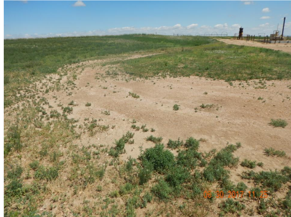
Photo 2: Photo taken from the well location, facing north. Photo shows access road loop leading to well has not been reclaimed and returned to crop.
