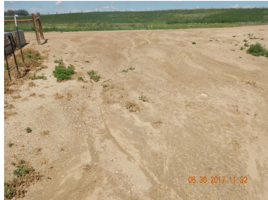
Photo 4: Photo taken from the battery, facing west. Photo shows erosion occurring on location.
