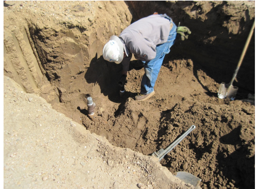
TAKE OUT RISERS OFF FLOWLINE HEATER AND HOOK UP DIRECT TO FLOWLINE ABBOTT12-21
