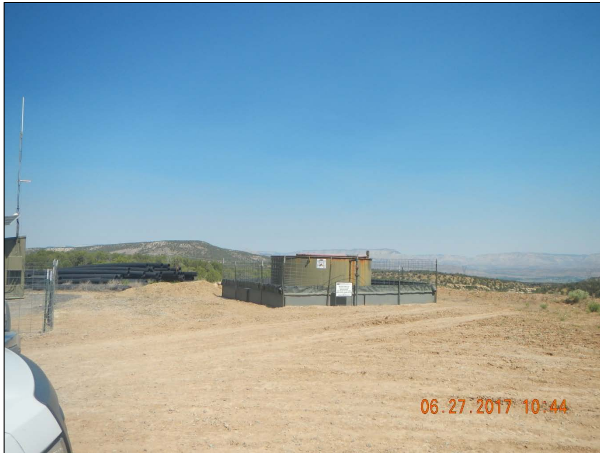
Tank battery and poly pipe stored on location.
