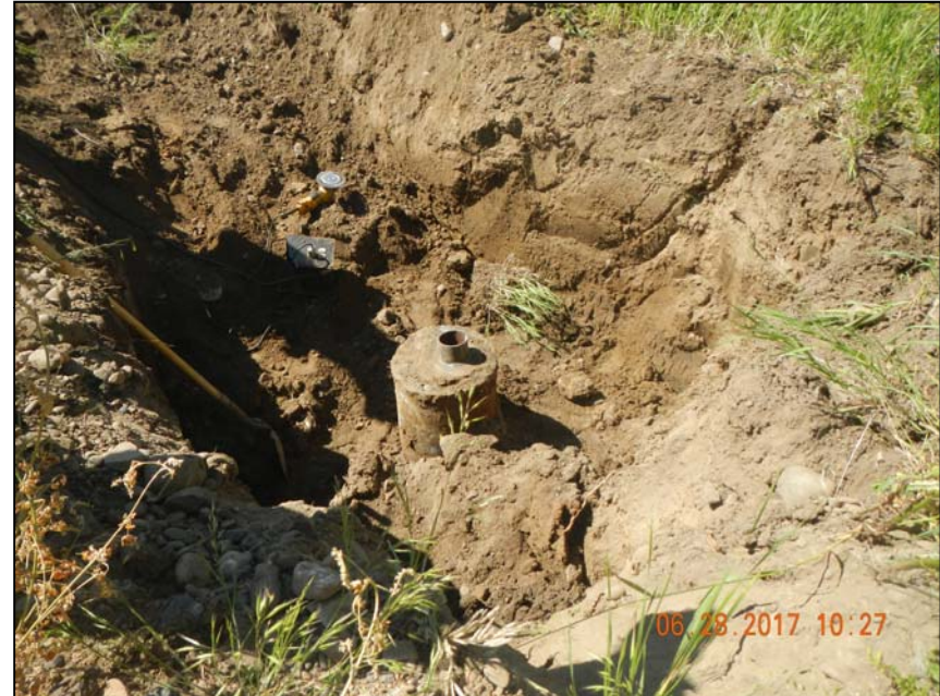
Photo 2. Above ground marker removed at surface casing.
