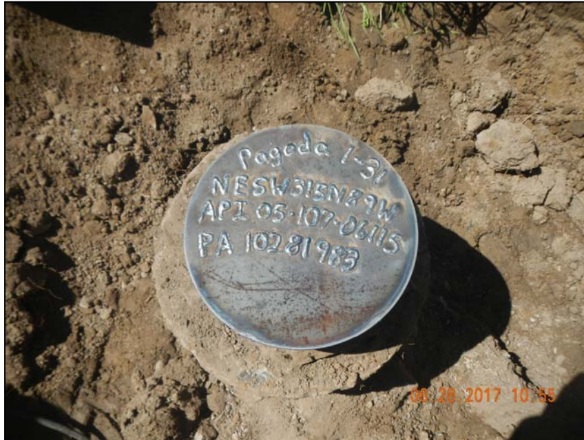
Photo 3. Below ground marker welded on at surface casing.
