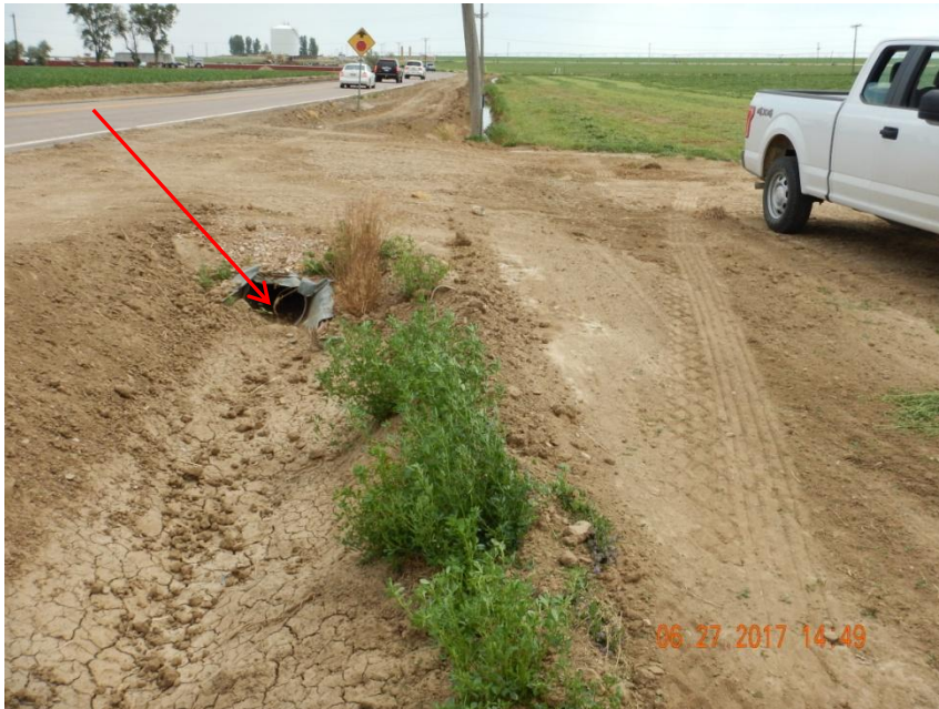
Photo 3. Photo taken from the entrance of the location, facing South. Culvert remains and needs to be removed per Rule 1004.
