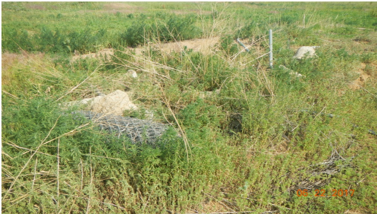
photo 6: There is cement blocks and fencing debris that remains at the location.
