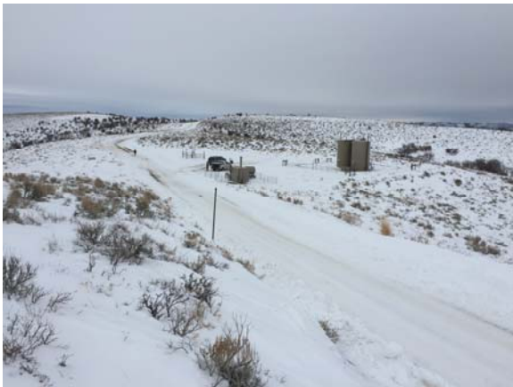
PAD OVERALL LOOKING NORTHERLY
