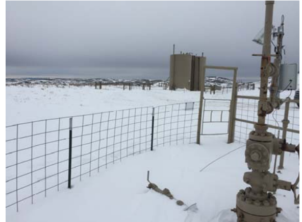
PAD LOCATION LOOKING SOUTH
