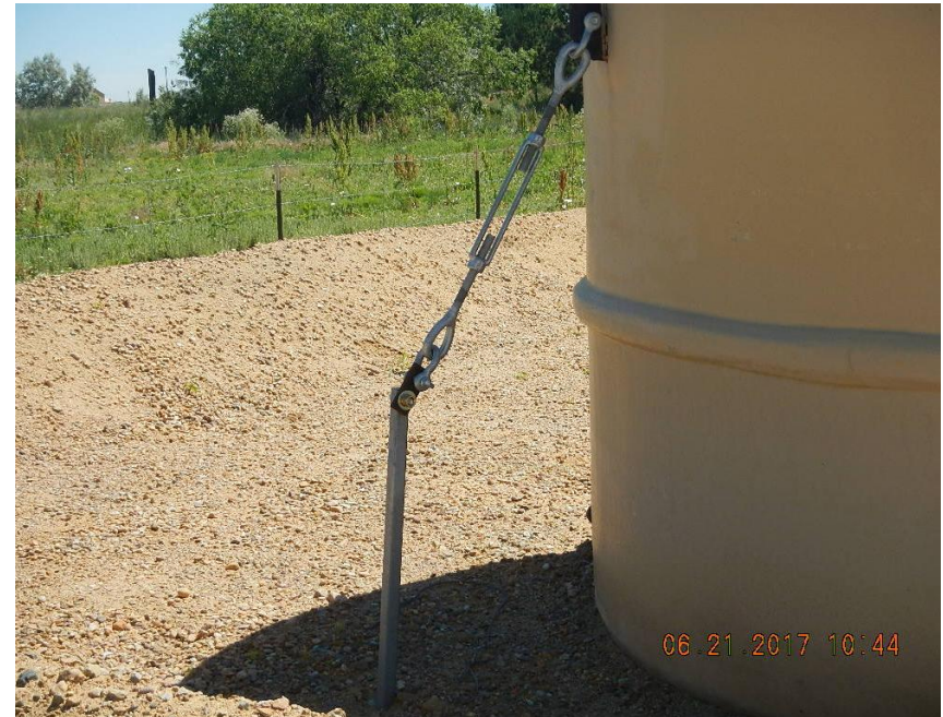
Photo 2 Flood anchoring on produced water tank (typical)
