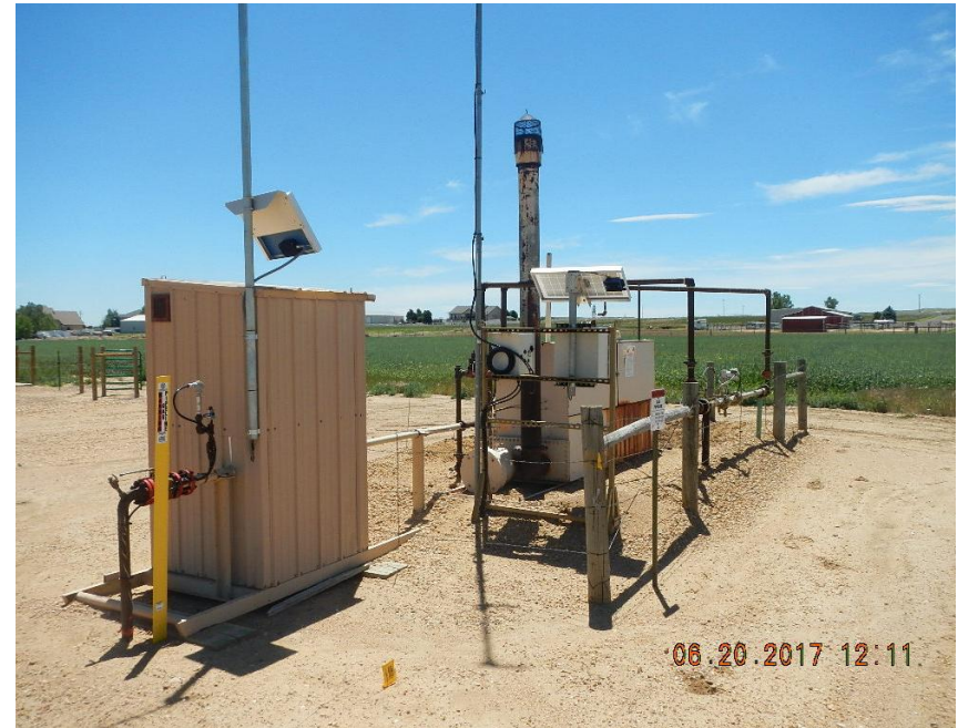
Photo 2 Separator and gas meter run from north
