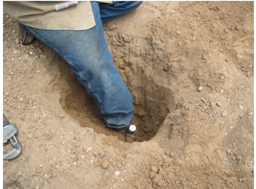
DIG UP AND PLUG 1" LINE AT ECD
