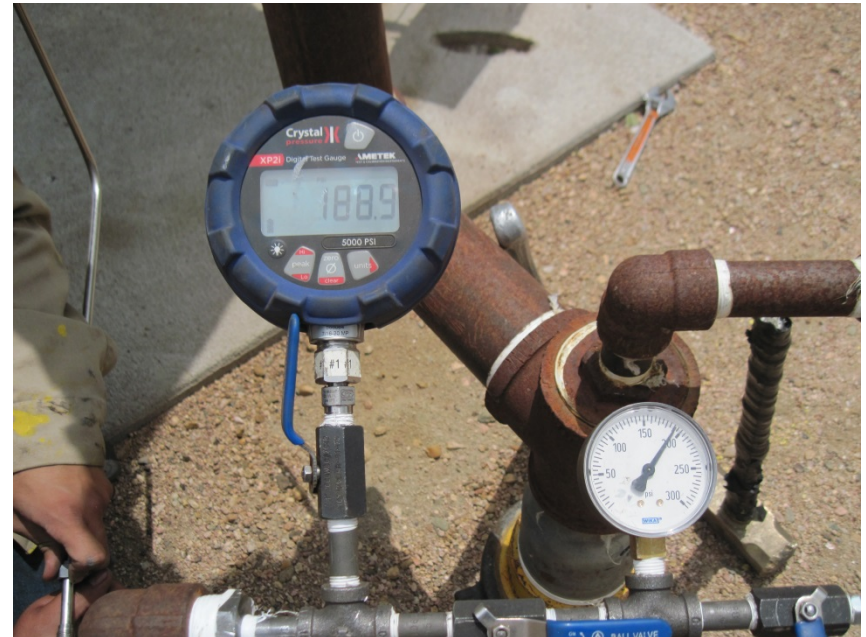
PRESSURE GAUGE AND RECORDER ECD 1" GAS BLOW DOWN LINE FROM SEPERATOR
