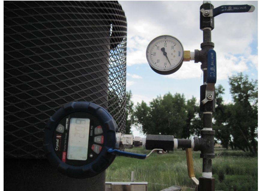
PRESSURE GAUGE AND RECORDER ECD 3" GAS LINE FROM PRODUCTION OIL TANK
