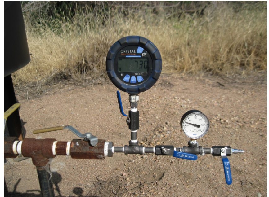
PRESSURE GAUGE AND RECORDER ECD'S 1" SUPPLY GAS LINE FROM SEPERATOR, BOTH 1" LINES
