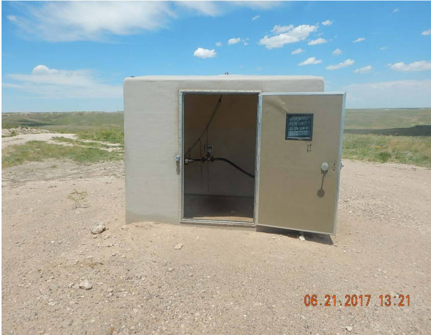
Photo 1: Wellhead, looking NW
