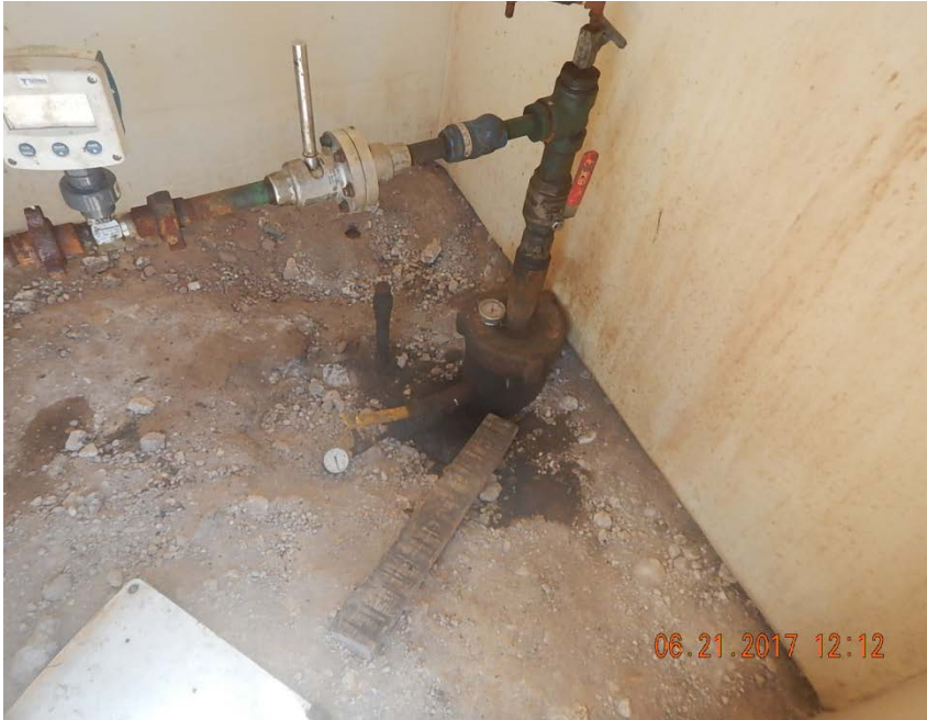
Photo 1: Stained soil at wellhead
