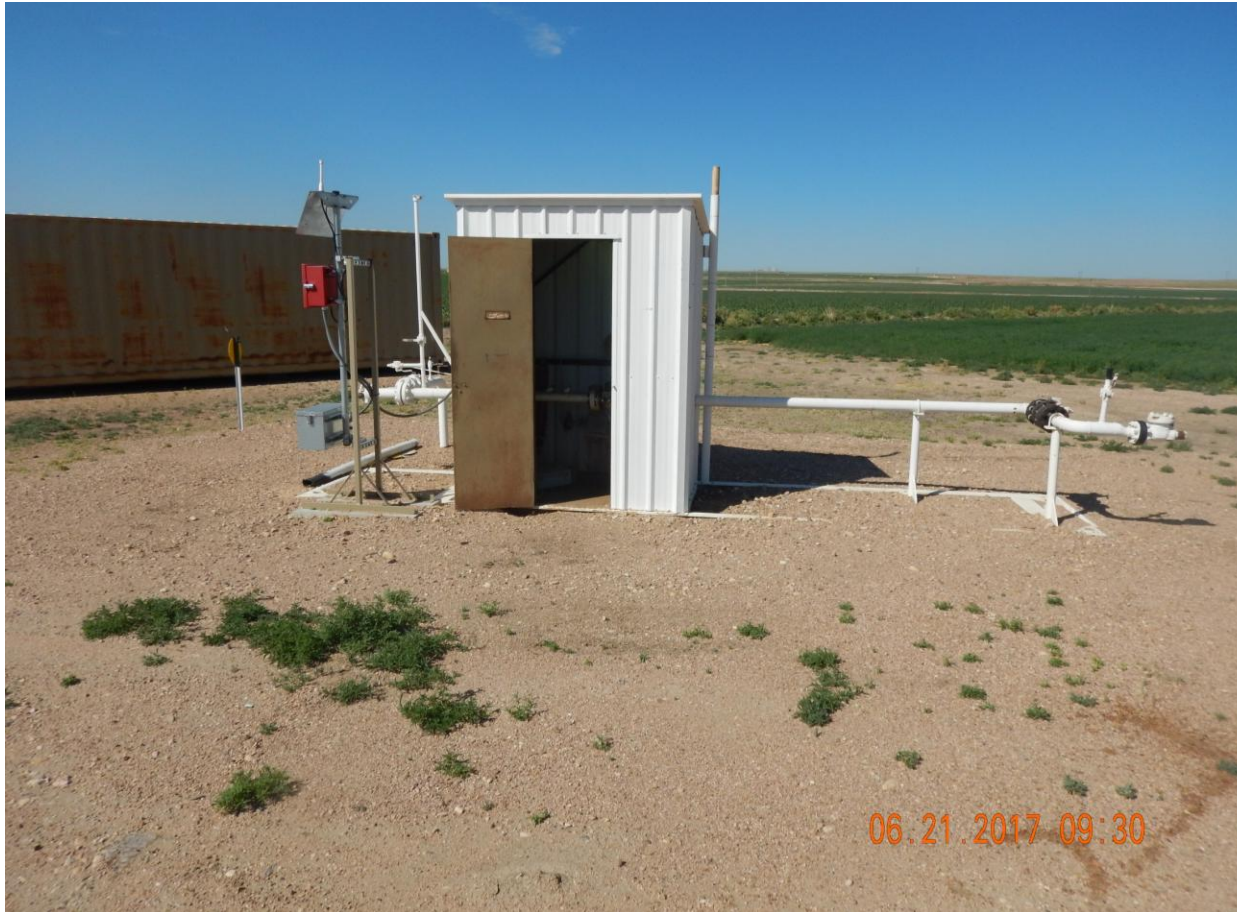
Photo 1: Photo taken from the well location. Photo shows meter shed still remaining on location.
