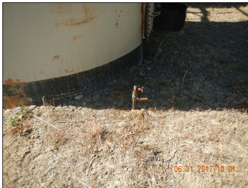
Photo 2. Unused riser not marked or locked out tagged out.
