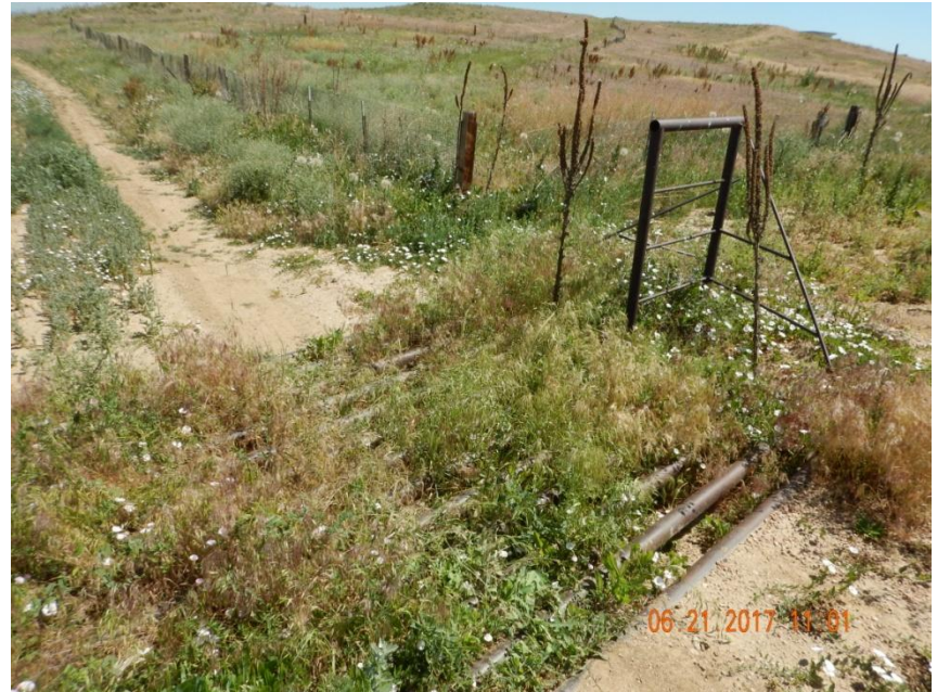
Photo 4. Photo taken from the just west of the meter shed, facing North. Operator needs to remove the cattle guard from location.
