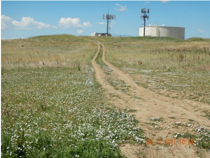
Photo 3. Photo taken from the well location, facing West. Access road has not been regraded and contoured per Rule 1004.
