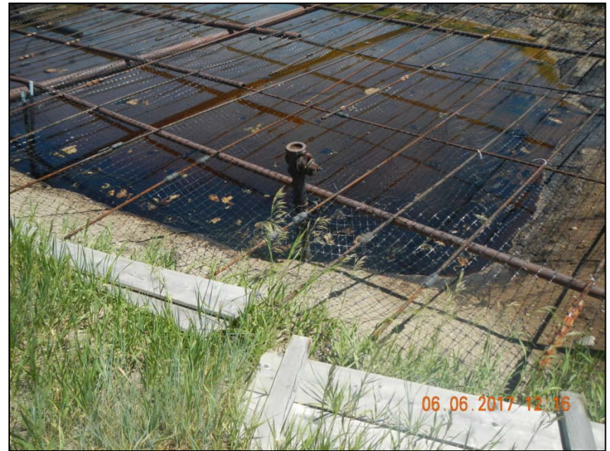
Photo 7. Pit with unused riser and sagging netting. Oil in pit.
