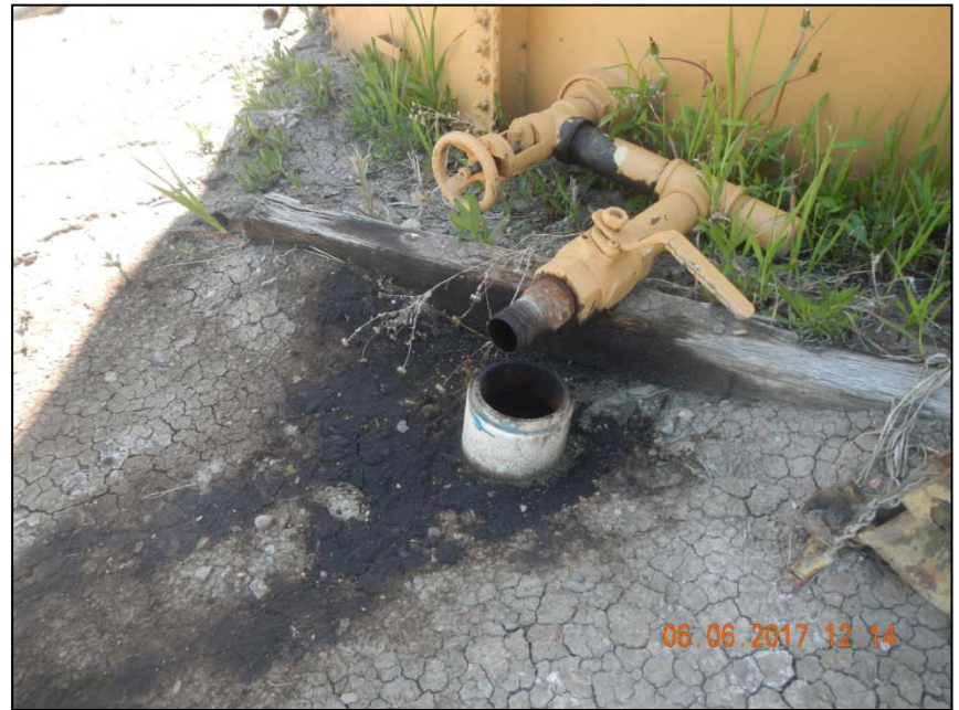
Photo 3. Stained soil at tank base.
