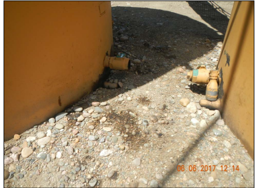
Photo 5. Stained soil at tank base.
