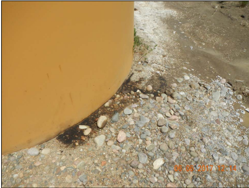
Photo 4. Stained soil at tank base.
