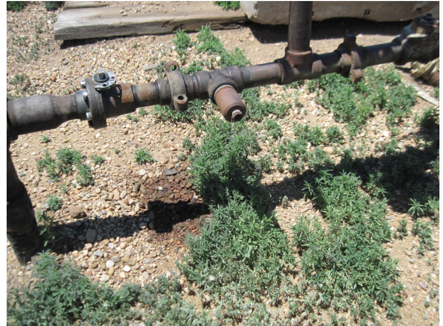
STAINED SOIL AT WELLHEAD
