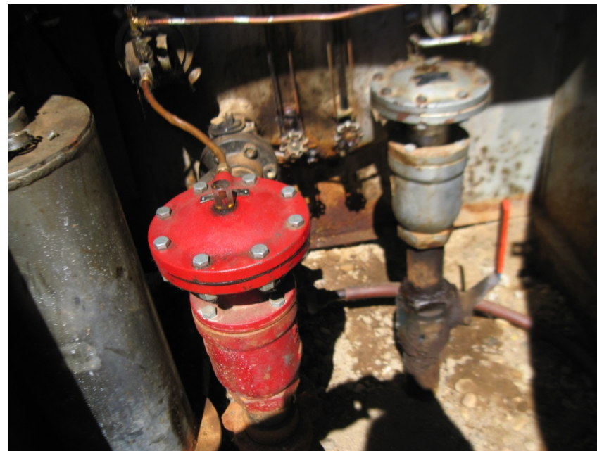
STAINED SOIL AND LEAKING PIPES INSDE SEPERATOR HOUSE
