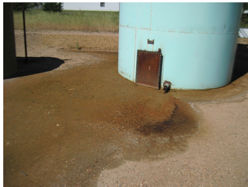
STAINED SOIL BEHIND OIL PROD TANK
