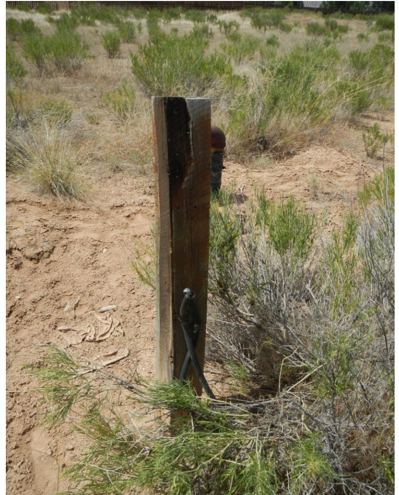
Photo#12: Wooden Post with electrical wiring remains .
