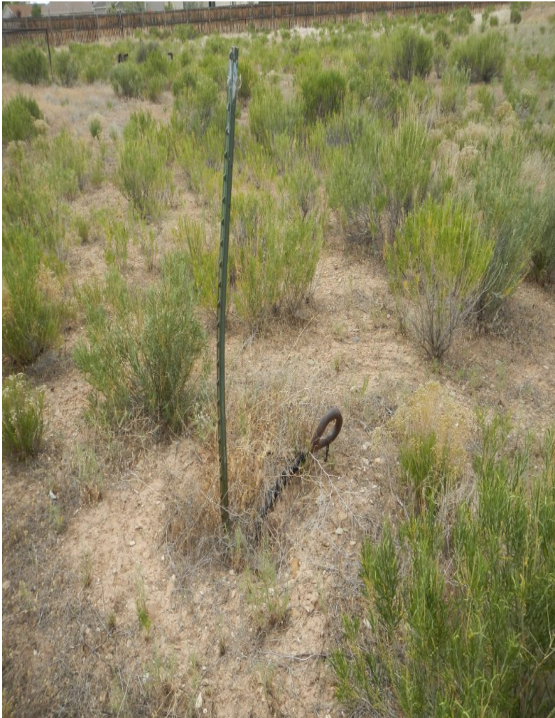
Photo#11: Guy Anchors remain .
