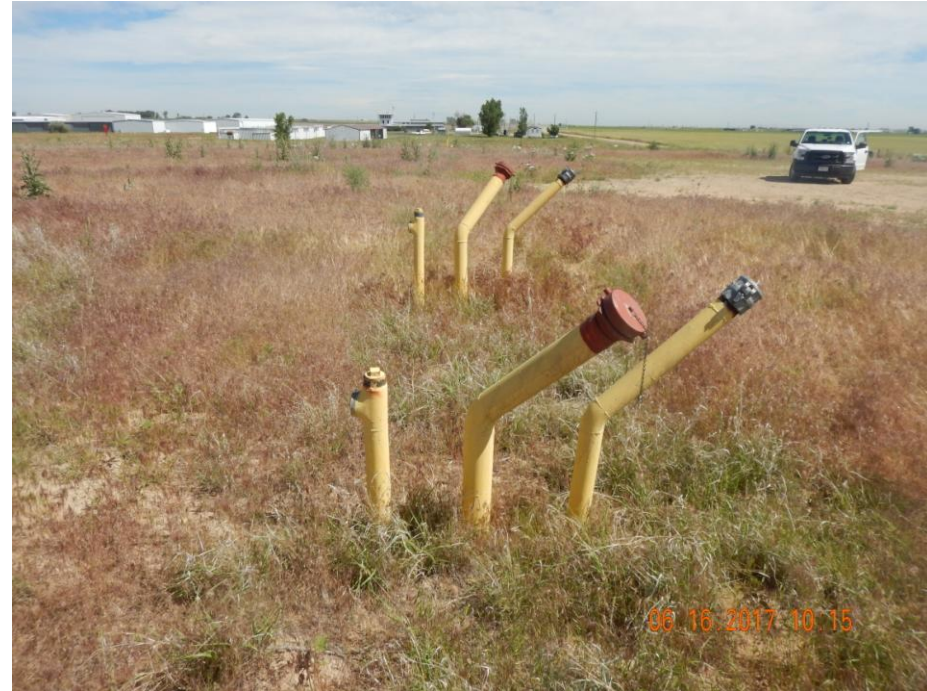
Photo 2: Photo taken from the west end of the battery location, facing north. Photo shows six pipe risers remaining at battery location.
