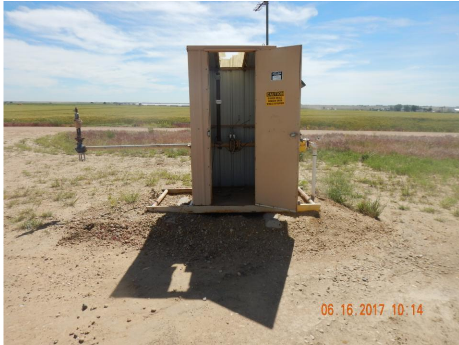
Photo 1: Photo taken from the battery location, facing east. Photo shows meter shed remaining at battery location.
