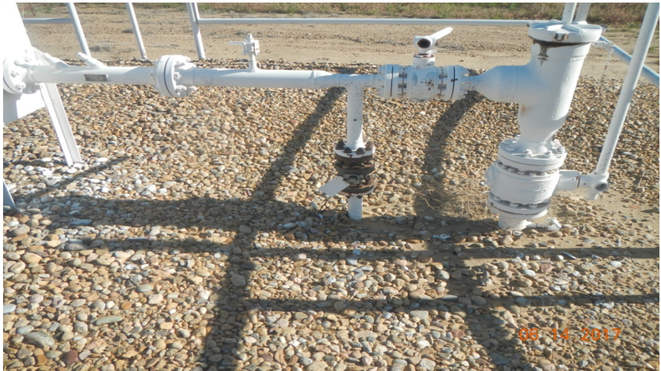
photo 2: The pipe infrastructure has valve handles that have not been locked and tagged out.
