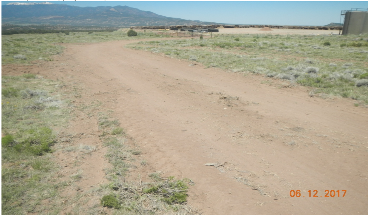
photo 8: Facing northeast toward the Freeman 3-24 location. A newly disturbed access road has been created that enters the west side of the location. No stormwater controls are in place.
