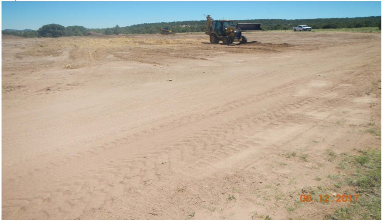
photo 4: Facing southeast toward the area of disturbance. The disturbed soils create a potential for wind erosion.
