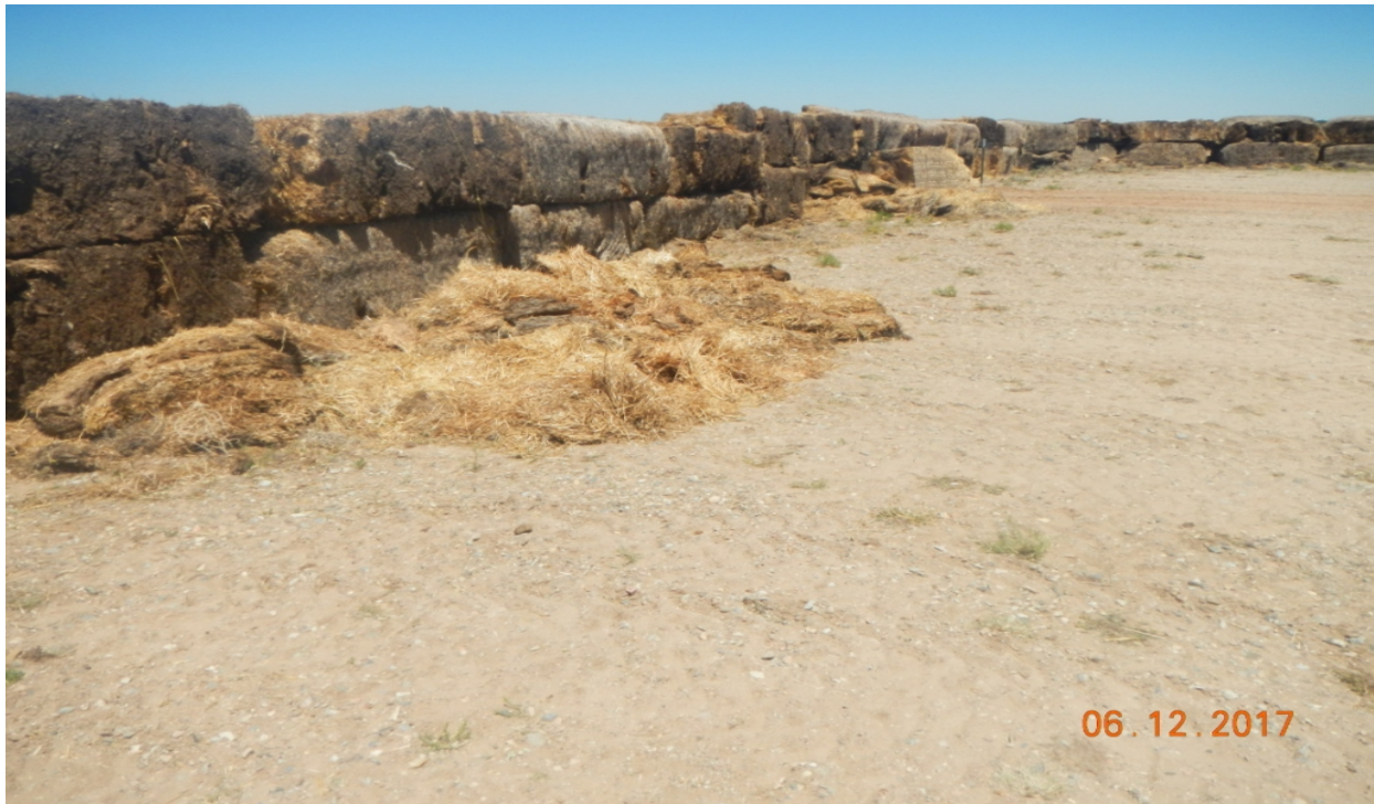
photo 13: The degraded bales remain around the north perimeter. The bales have been staked since the previous inspection and many have fallen apart.
