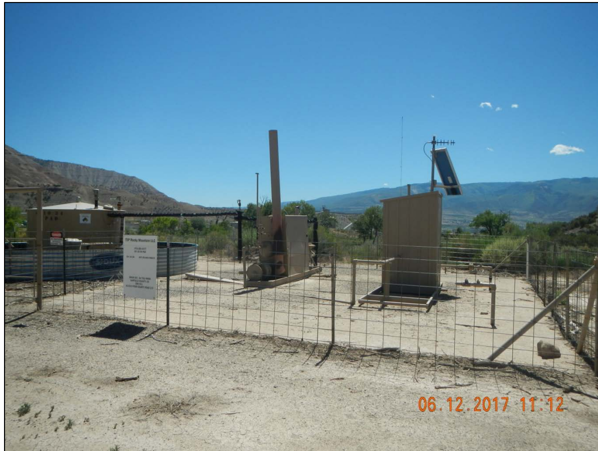
Tank battery, meter house, and separator.
