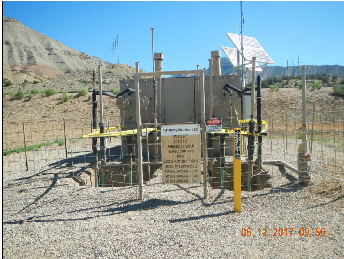
Separators: Unused flowline being plugged and capped.
