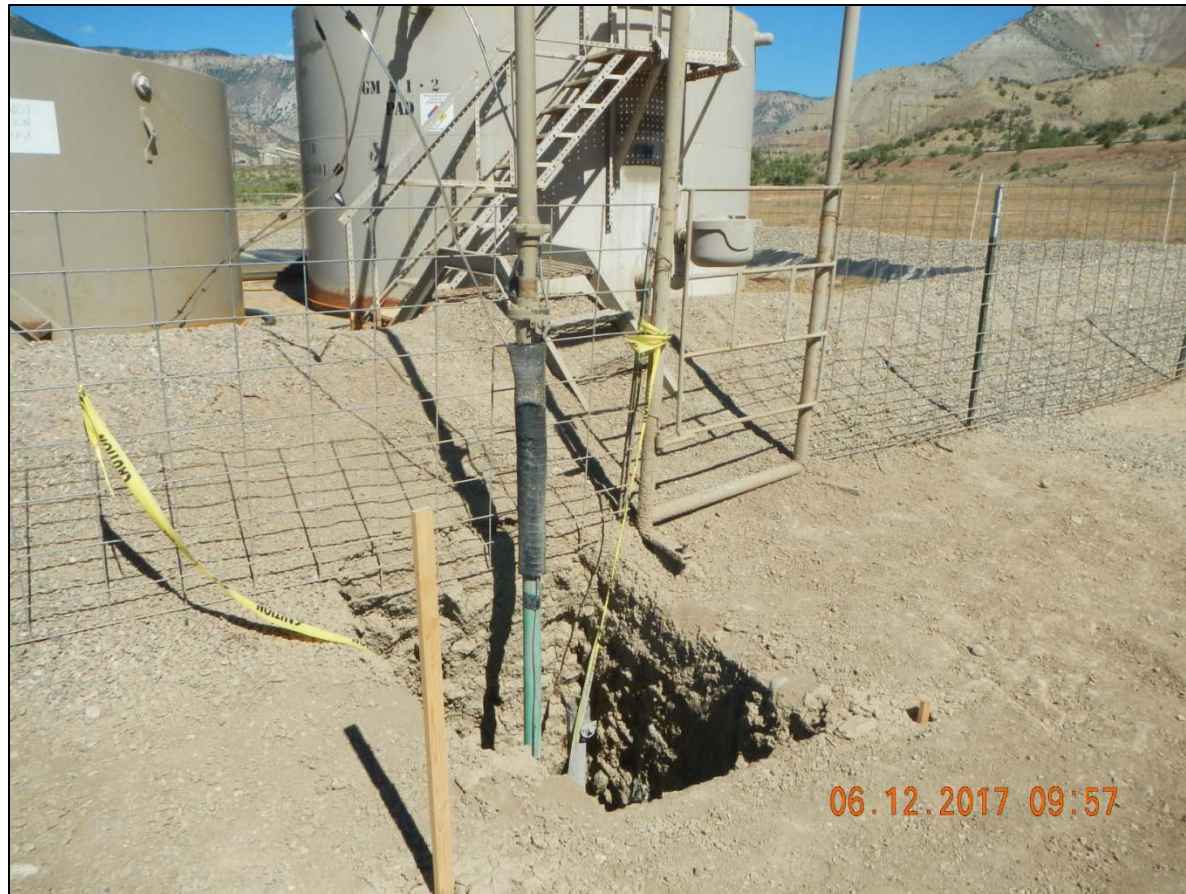
Tank battery: : Unused flowline being plugged and capped.
