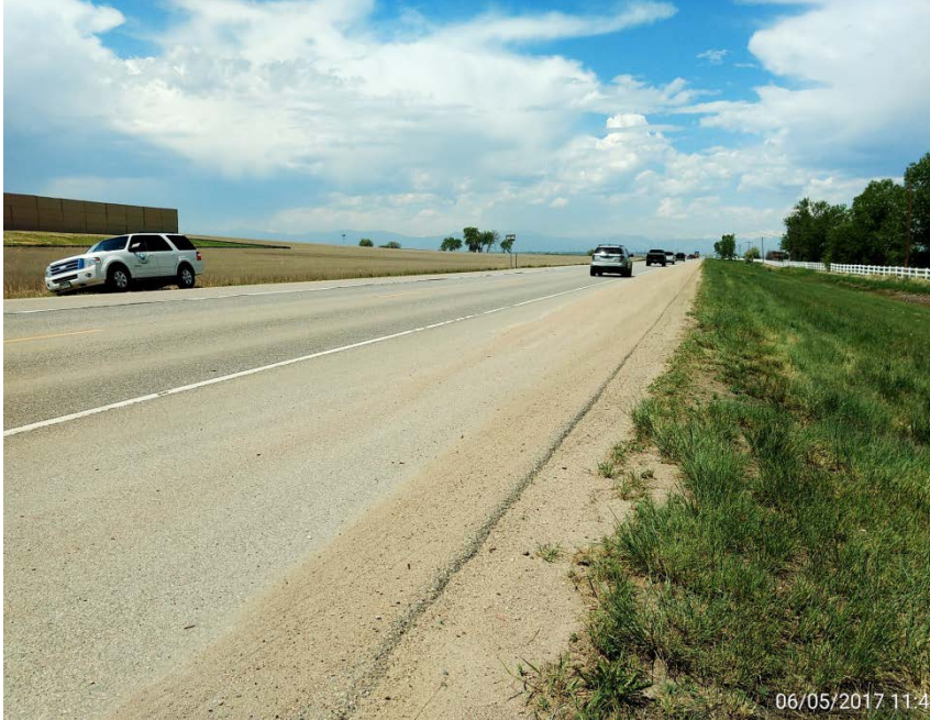
Photo 3: Stormwater tracking on Highway 7, looking W
