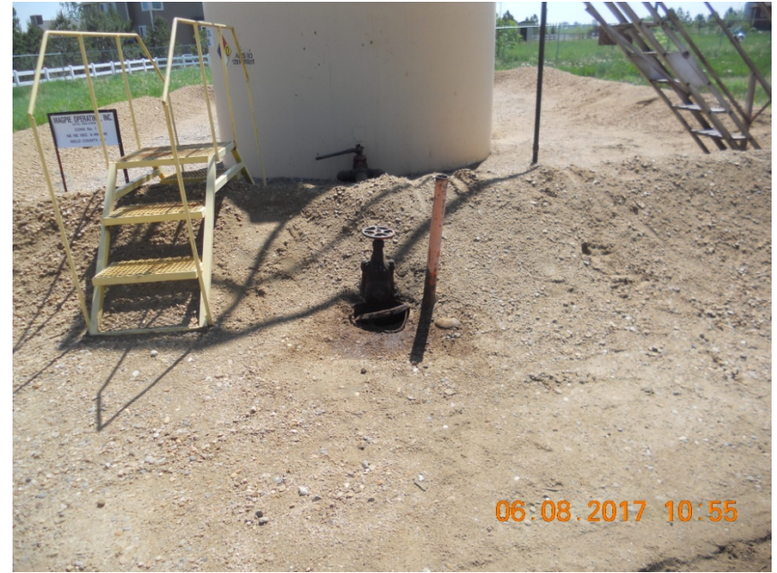
Photo 12. Spillage at loadline
