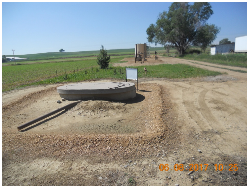
Photo 5. Battery looking south from north end of water vault. Note lack of secondary containment .
