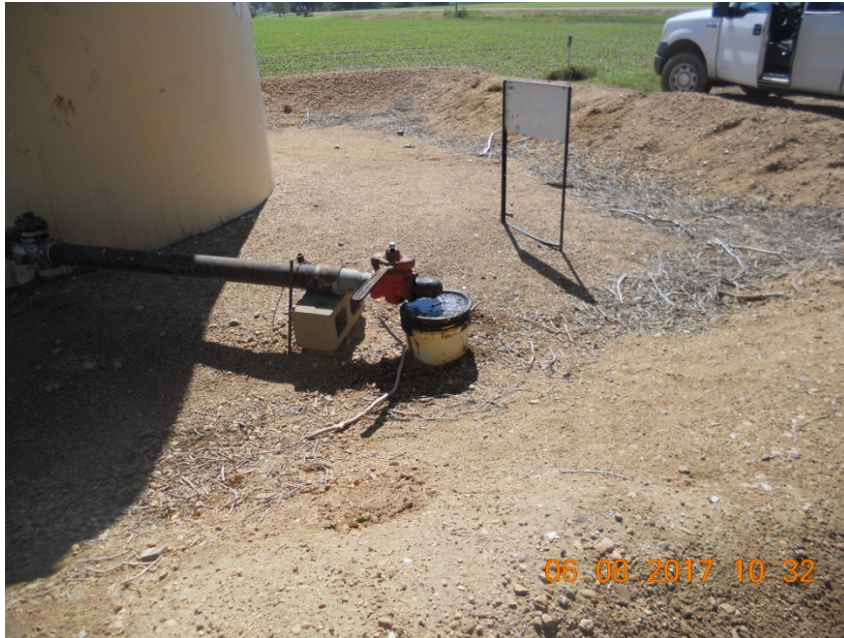
Photo 3. Containment device full
