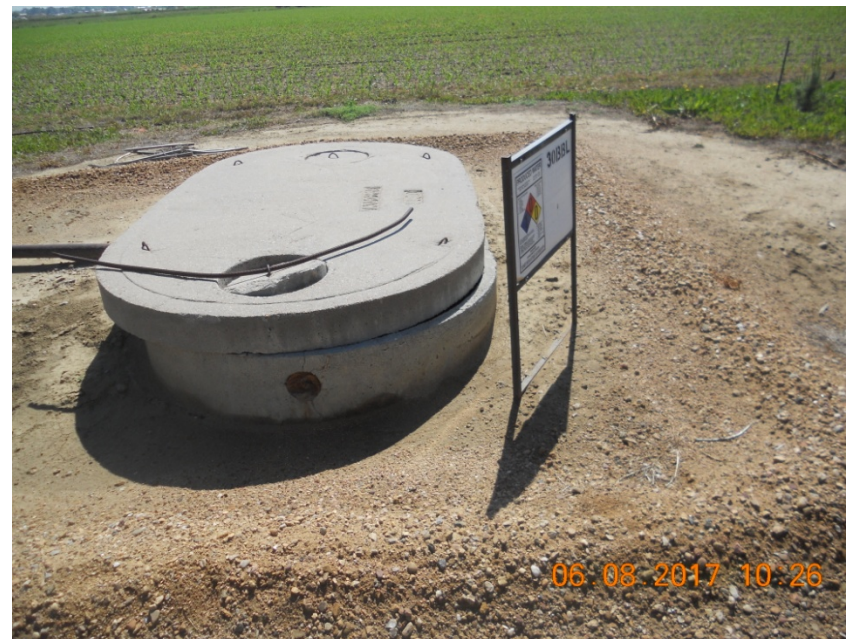
Photo 6. Water vault lid moved over. Note lack of secondary containment .
