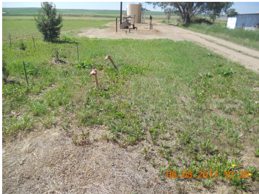
Photo 7. Looking south from water vault. 2-2" risers not marked not locked out tagged out.
