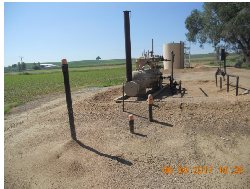
Photo 8. Unused 3-3" & 1-2" risers north of separator
